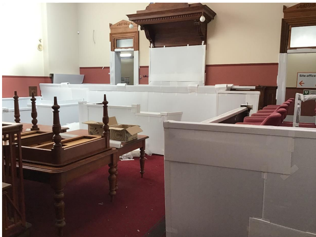
Photo 16: View of Main Courtroom showing protection of timber elements
