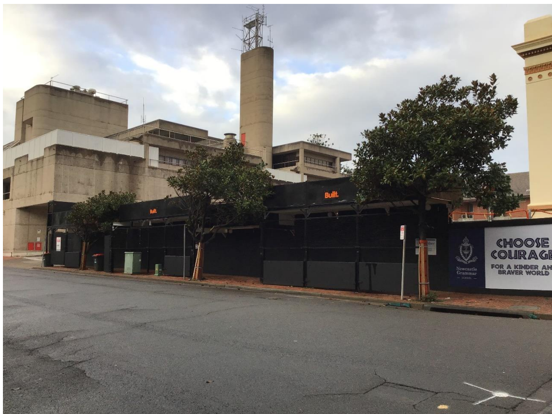
Photo 08: View from Church Street of B-Class Hoarding & Building A area.
