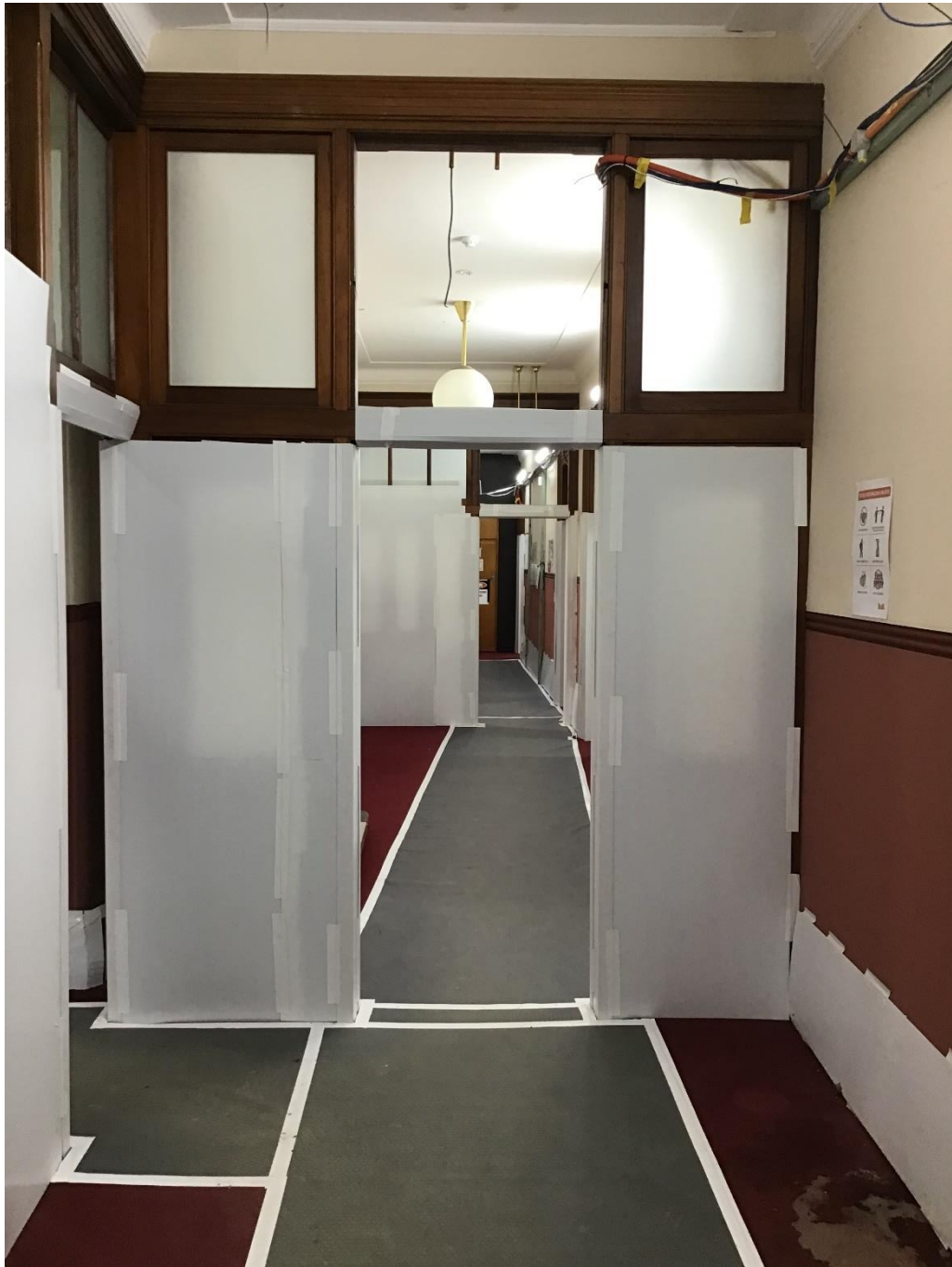
Photo 17: View of Corridor showing protection of doorways and timber elements. Doors have been removed and carefully stored for reinstatement
