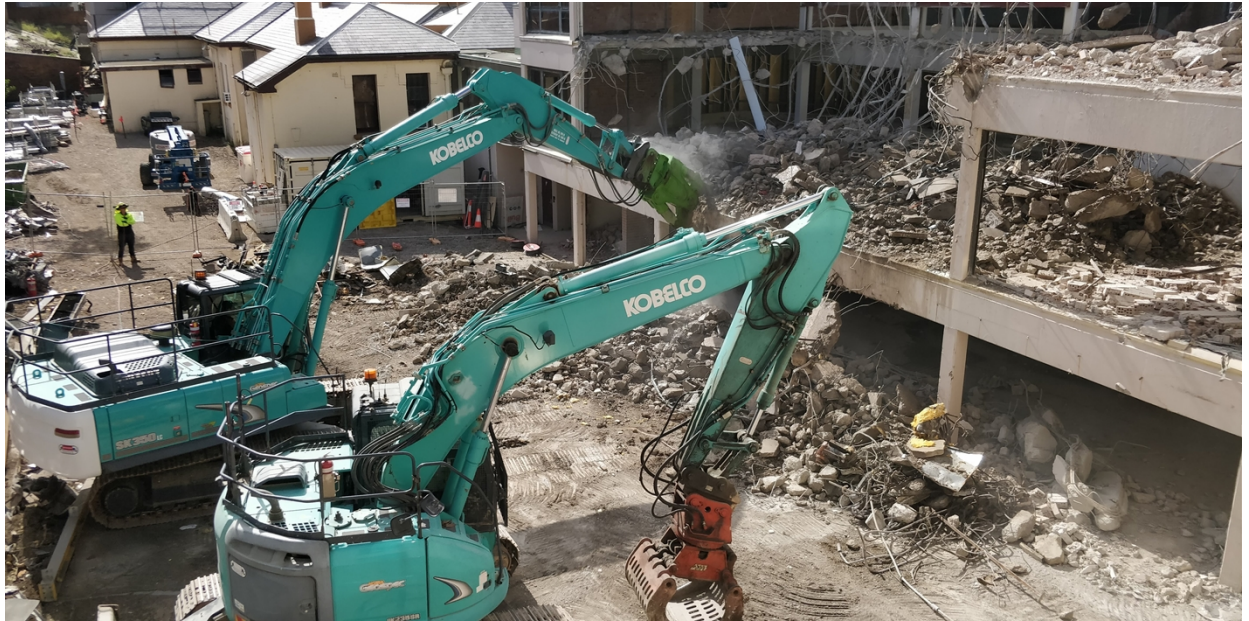
Figure 2 Site Demolition Operations
