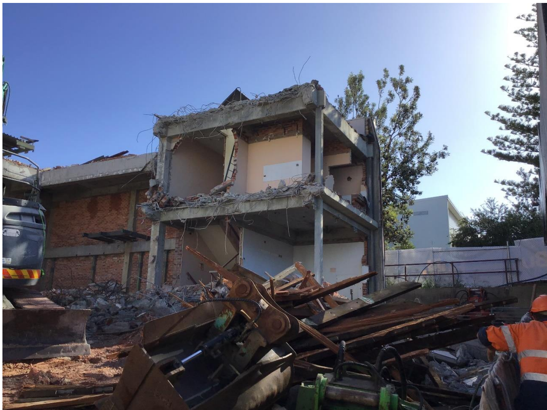
Photo 10: View from Building C Vehicle Gate looking West showing structural demolition of Supreme Court Building
