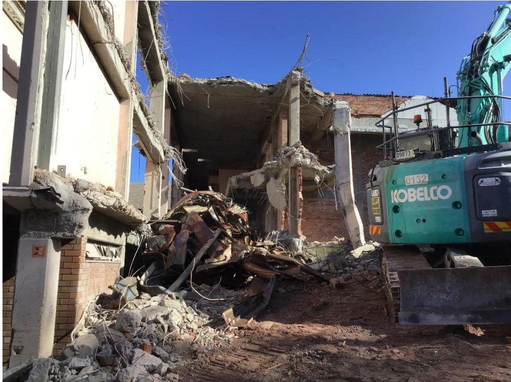
Photo 11: View from Building C Vehicle Gate looking South showing structural demolition of Supreme Court Building
