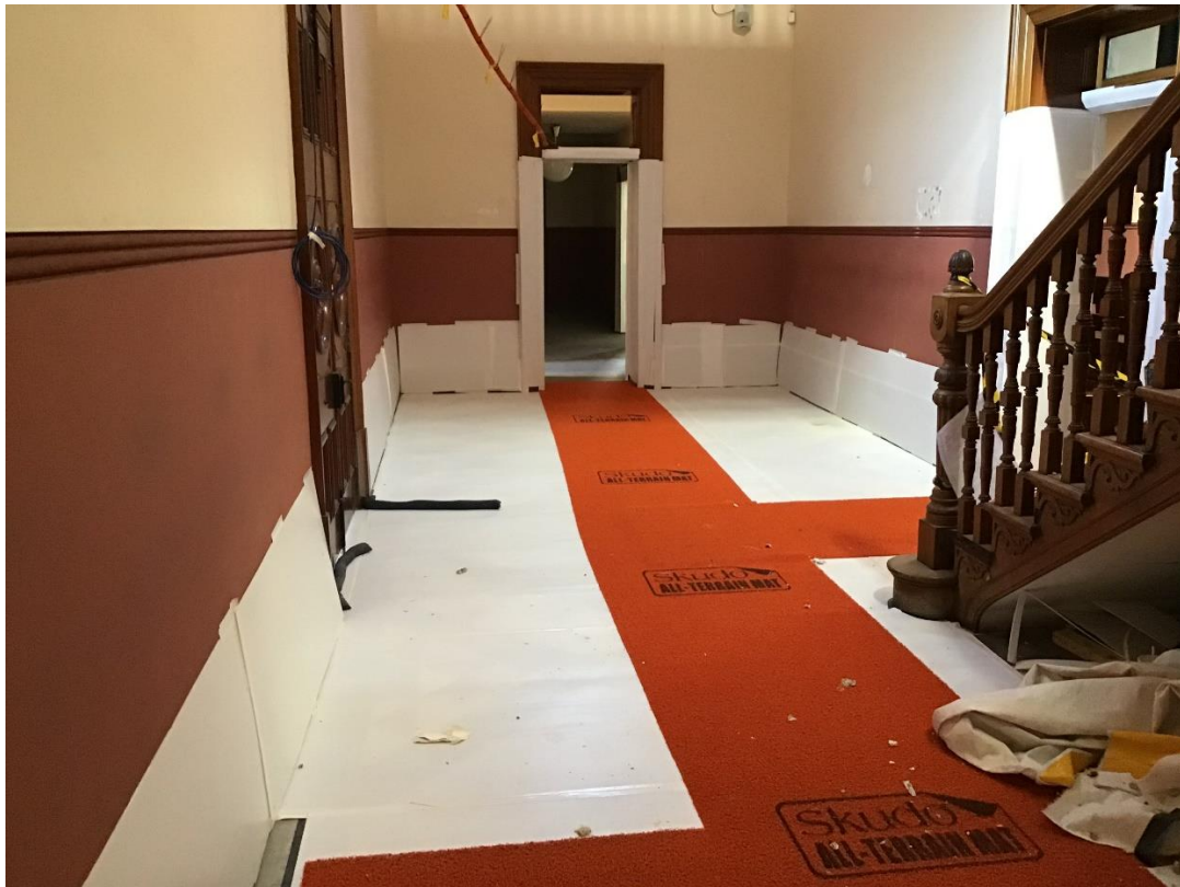
Photo 15: View of Heritage Building Foyer showing protection of tiles and timber elements
