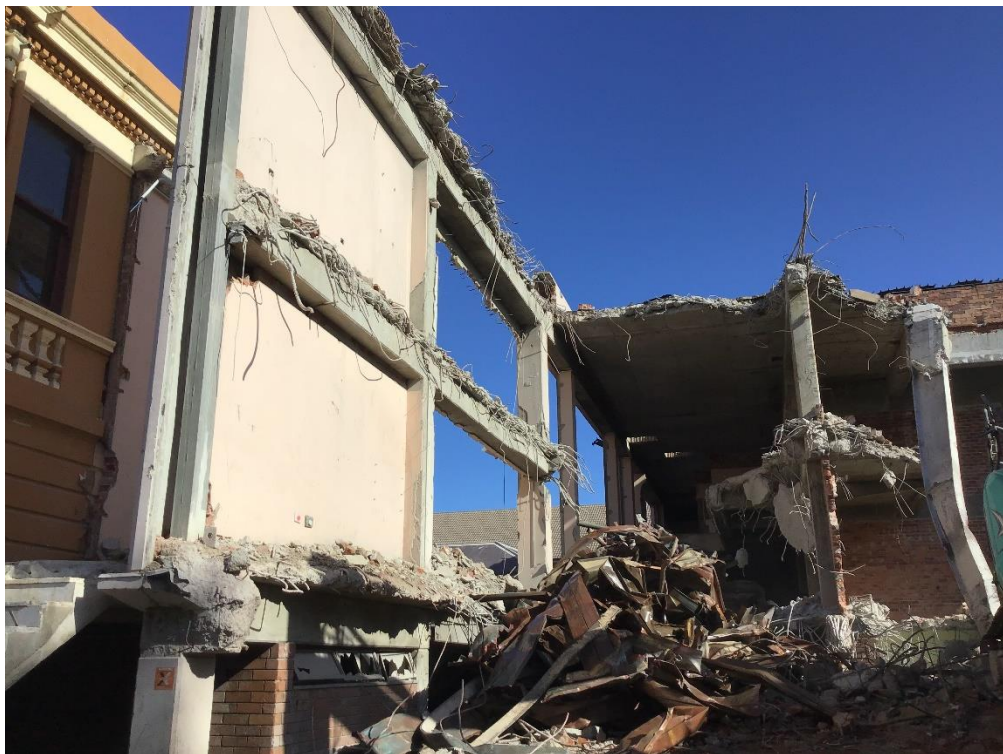
Photo 12: Photo looking South-East showing Building B & C connection demolished
