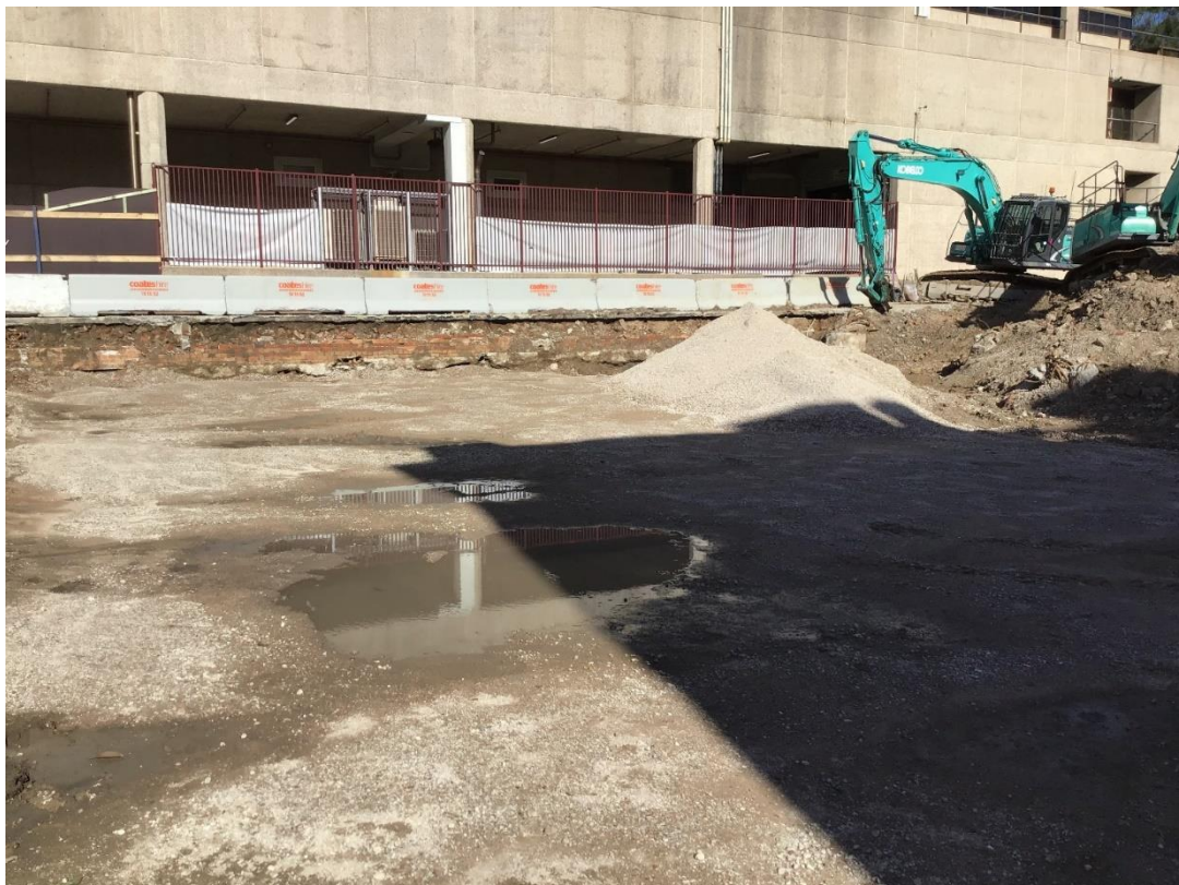
Photo 21: View from front of compacted section of Building A looking East
