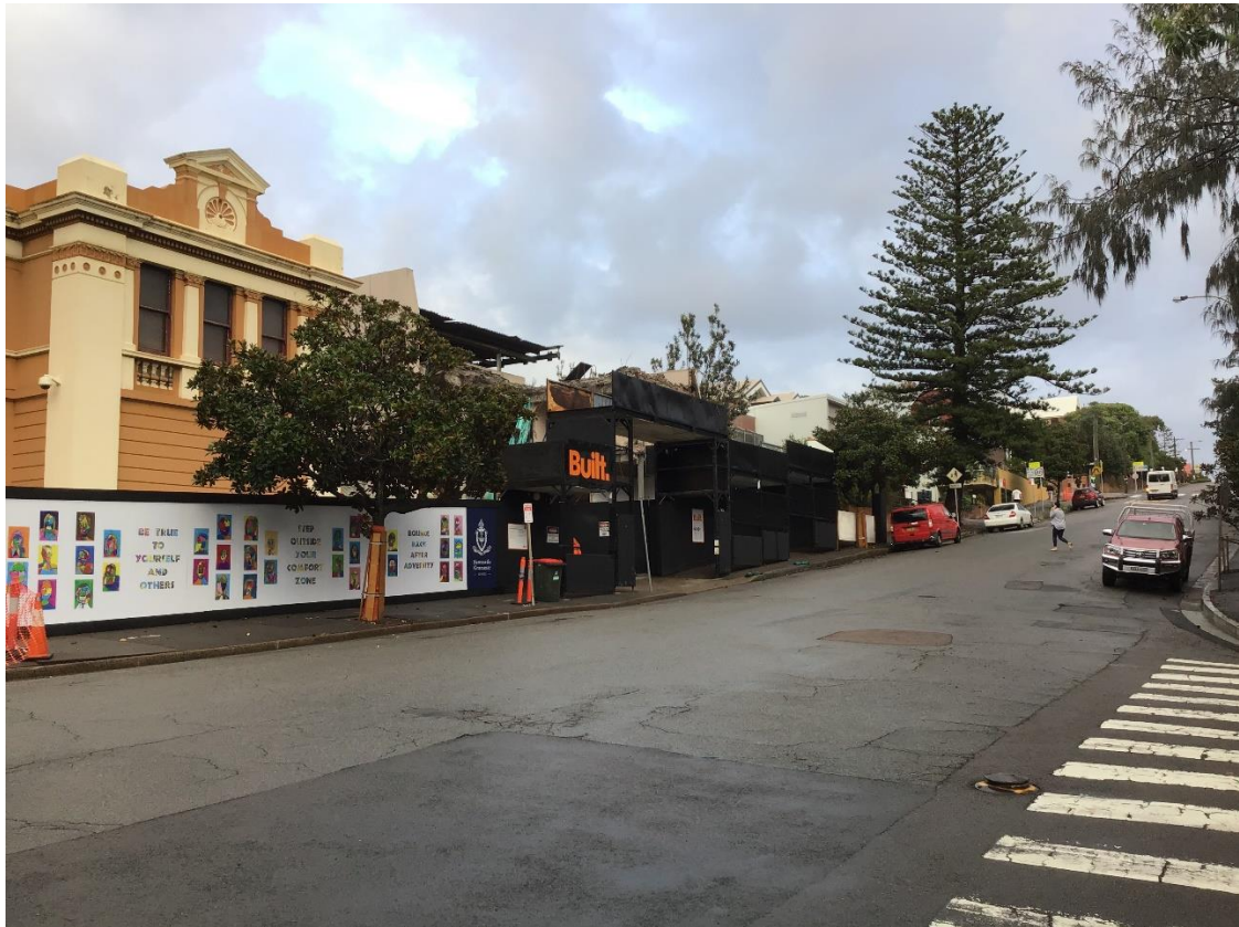
Photo 07: View from corner of Church & Bolton Street looking South-West showing Building C, B-Class Hoarding & Vehicle Gate
