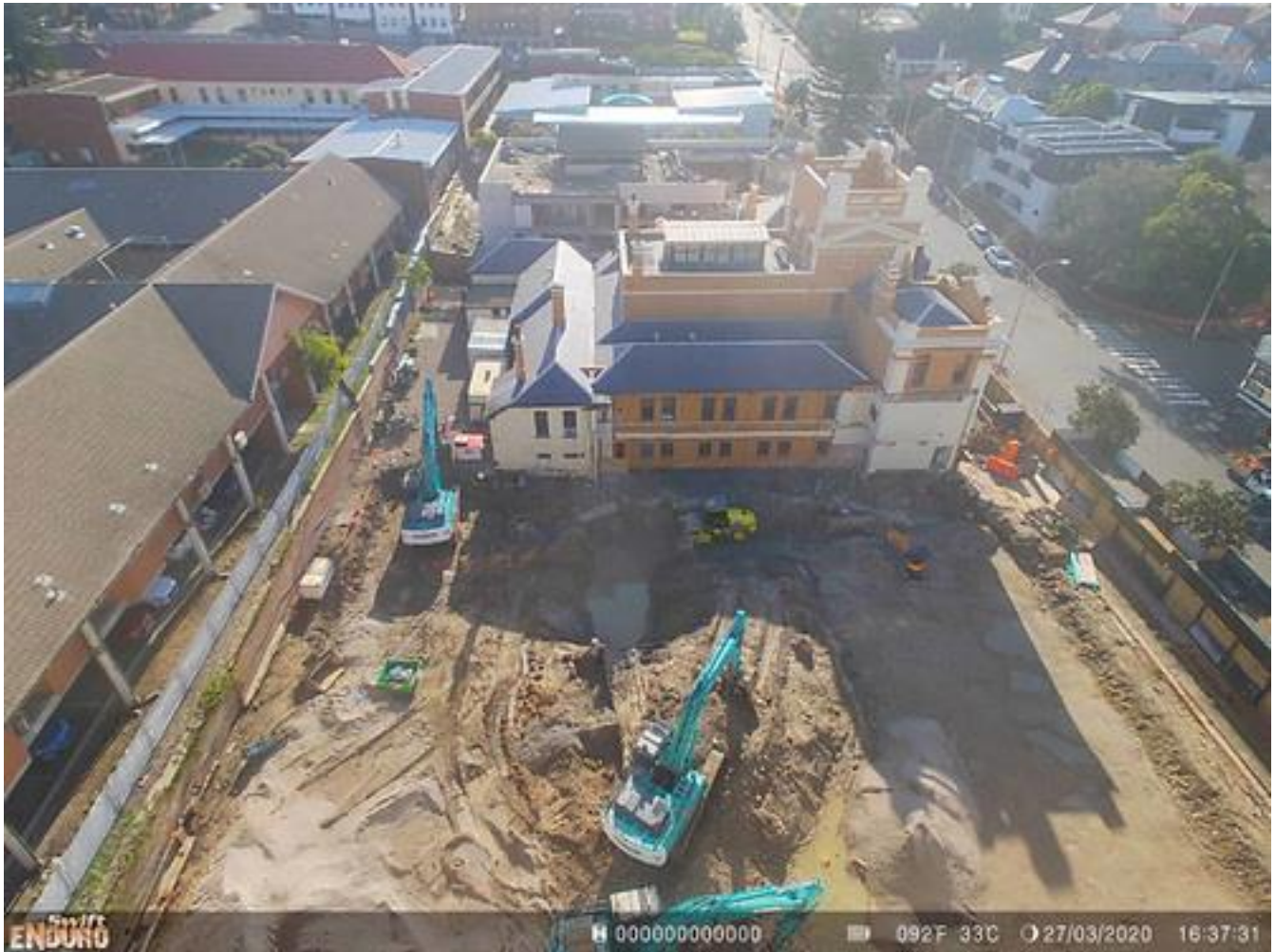
Photo 02: Time-lapse photo of the site taken on 27/03/2020
