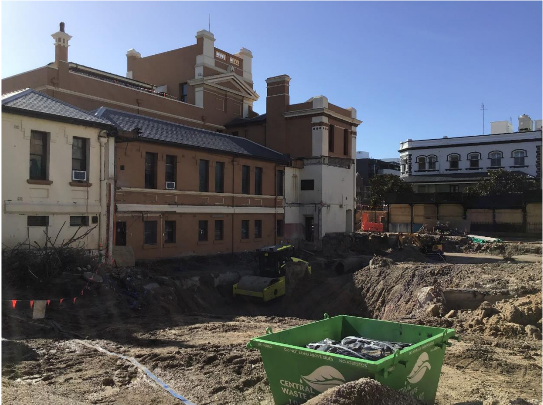
Photo 18: View from rear of Building A looking North-West showing extent of earthworks
