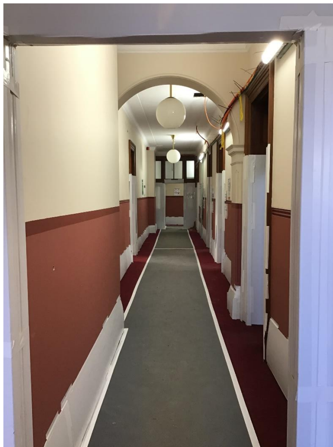
Photo 14: View from Heritage Courthouse Entry showing protection of timber elements
