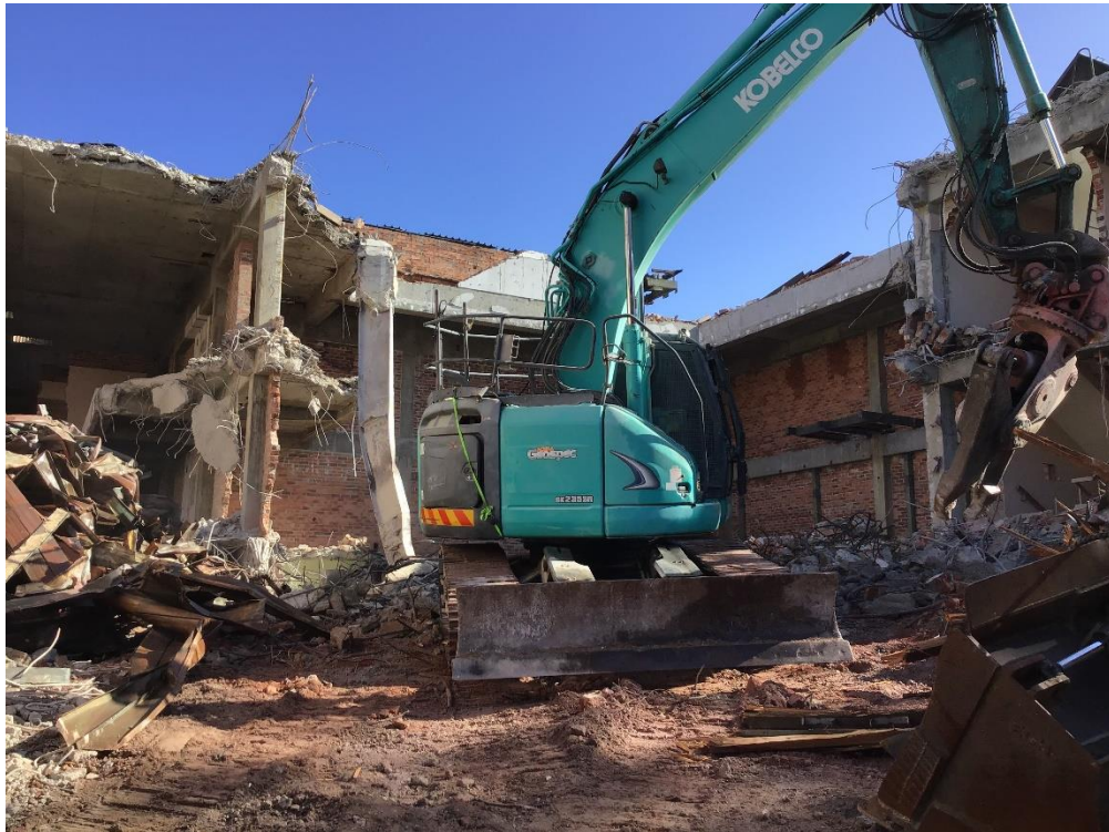
Photo 13: View of excavator with shears used for structural demolition in Supreme Court Building
