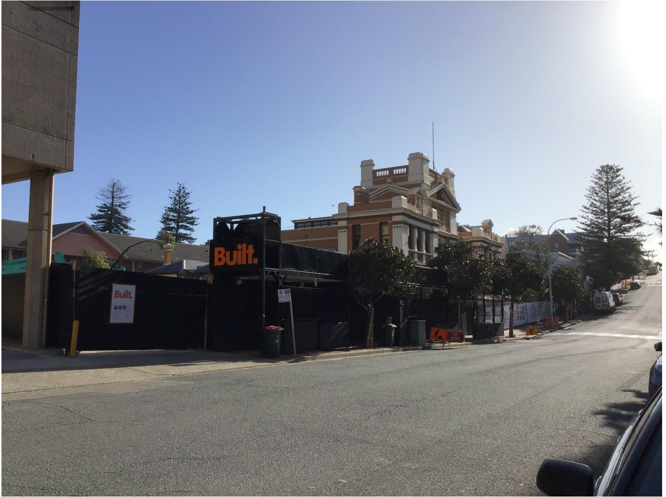
Photo 03: View of site from Church Street facing South-West showing B-Class Hoarding, Vehicle Gate & Work Zone
