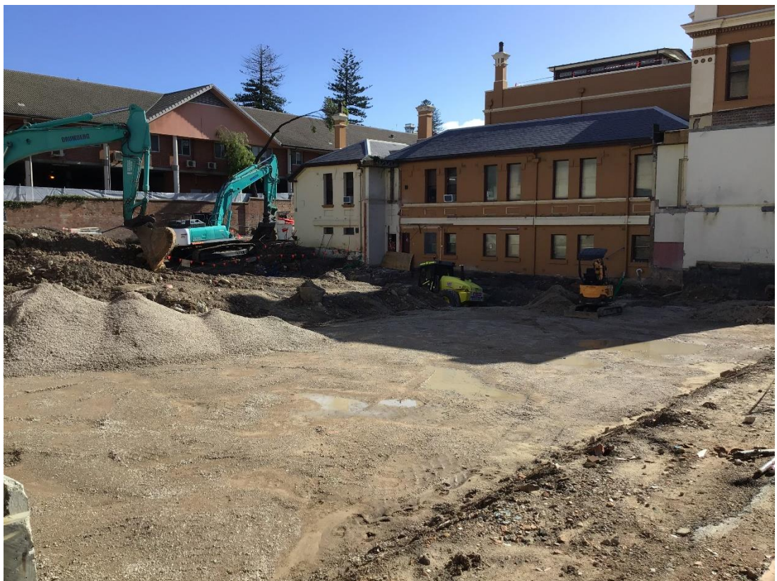
Photo 19: View from front of Building A looking South-West showing imported compacted fill.
