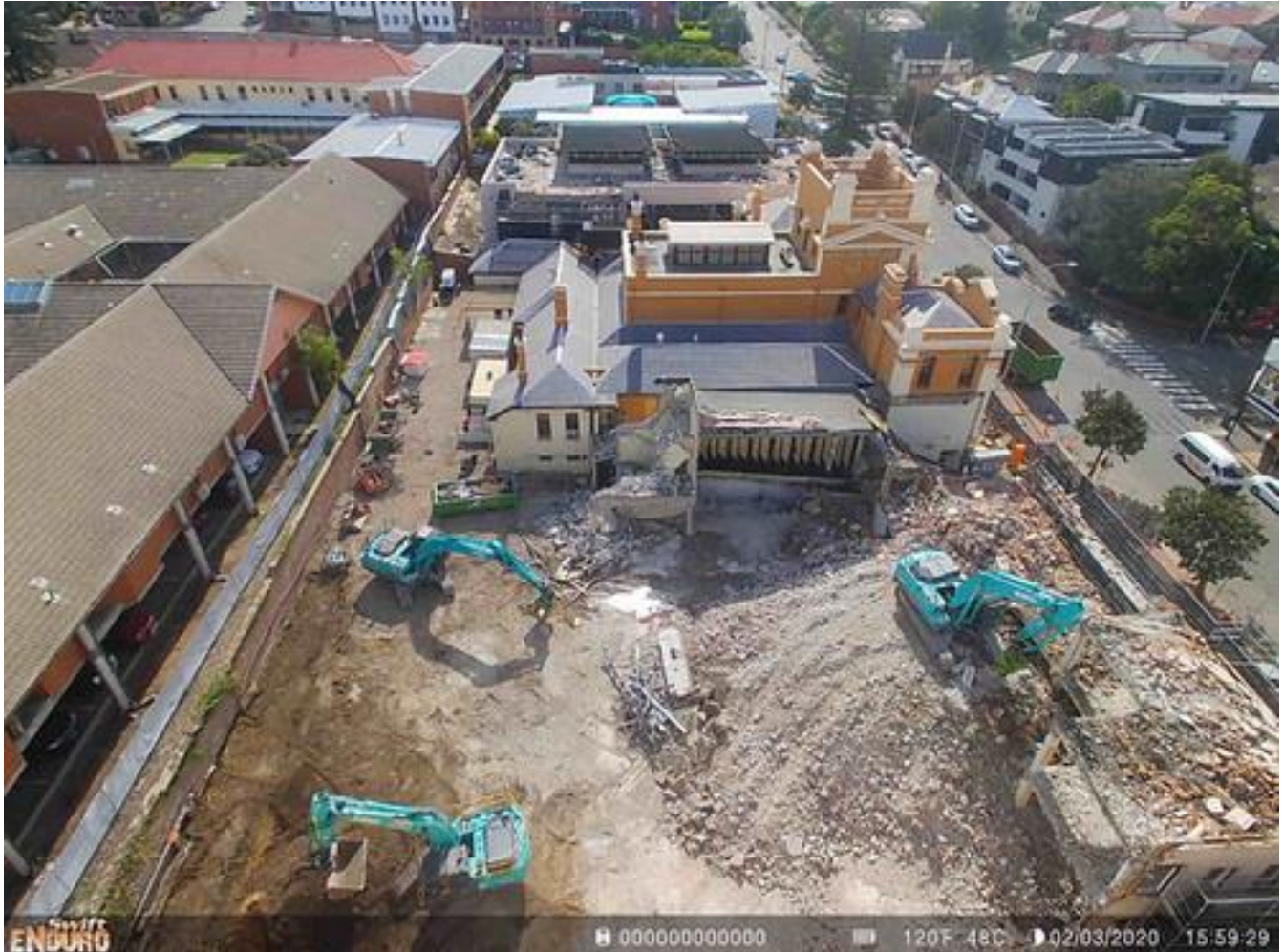
Photo 01: Time-lapse photo of the site taken on 02/03/2020
