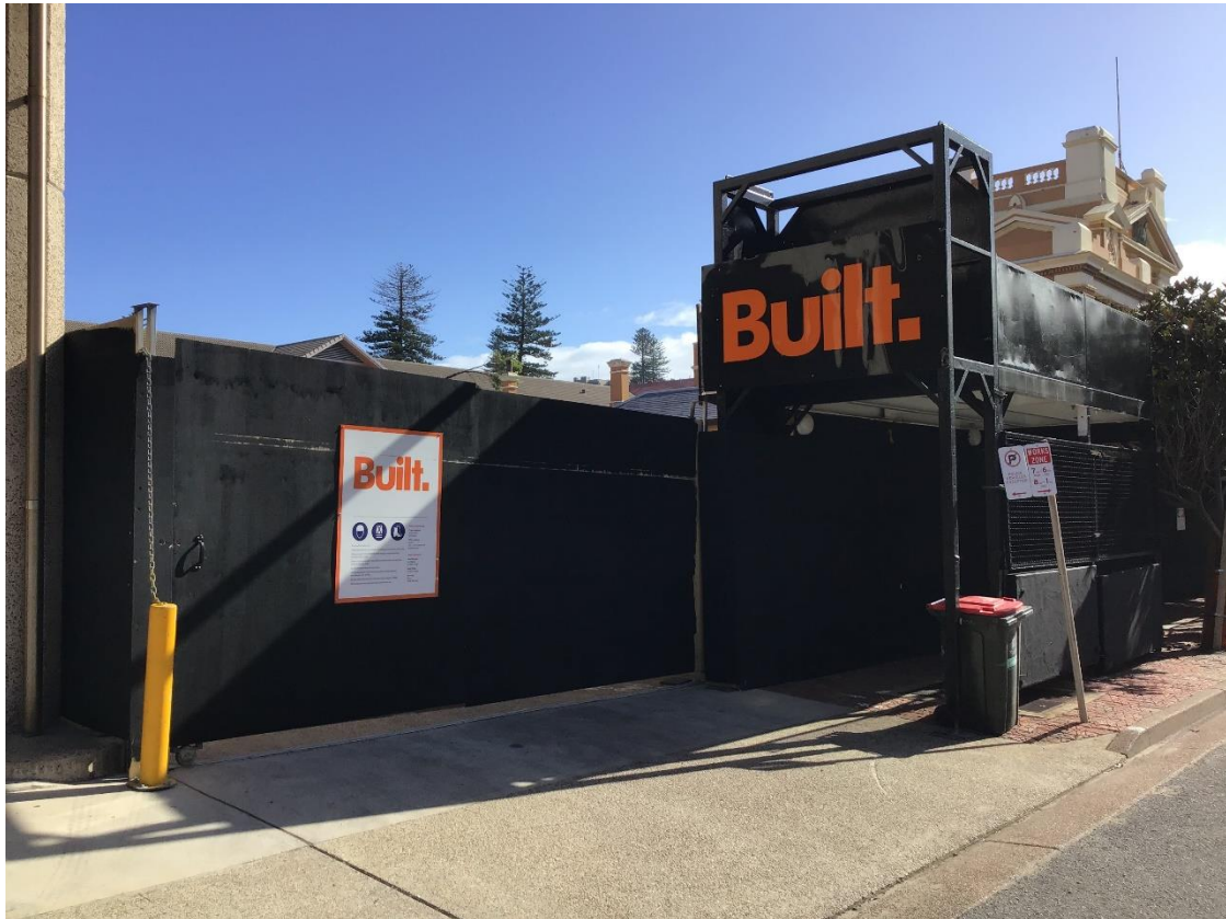
Photo 09: Building A Vehicle Gate & Hoarding/Gantry
